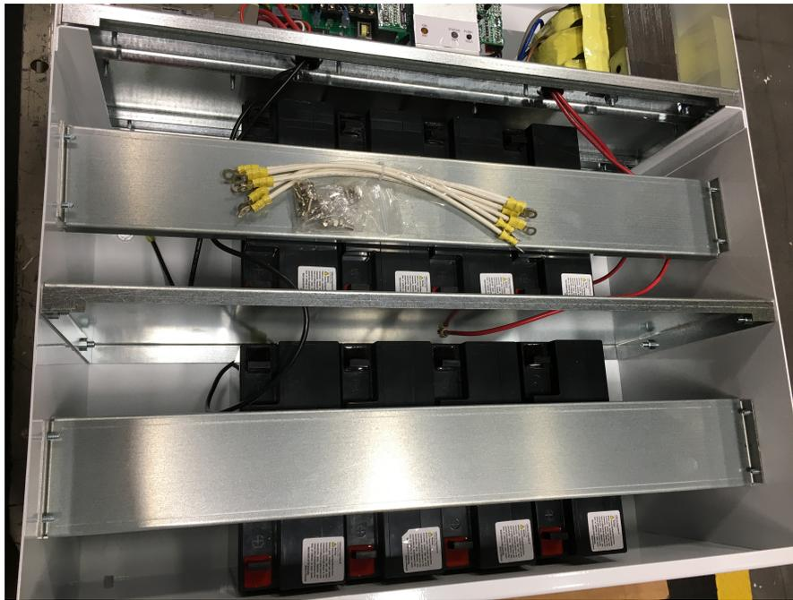
*Battery retention brackets installed on the front*
