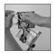
2. Make AC wiring connections to Base Plate Assembly with standard wire nuts. BLACK: 120/277 VAC Universal Input
