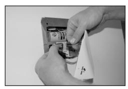
4. Connect polarized plugs for Test Panel and LED lamps. NOTE: IF AC BUILDING POWER IS NOT SUPPLIED, THE FIXTURE WILL OPERATE IN EMERGENCY MODE. TO MINIMIZE BATTERY DISCHARGE, TURN AC POWER ON WHEN WIRING CONNECTIONS ARE COMPLETE.
