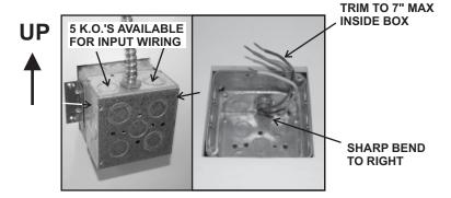
1. Install standard 4" x 4" x 2 1/8" DEEP J-box, together with 1 ½" extension ring. AC power input wiring can be routed through 5 KO locations in lower J-Box, as shown above. TRIM AC INPUT WIRING TO LENGTH AND SHAPE AS SHOWN
